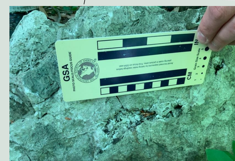
Figure A. Damage zone rock located near the east entrance of the Broomstick Ledges
